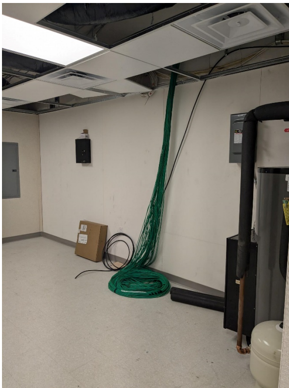
Fiber cable installation
