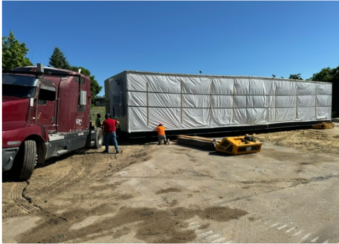
Southside Modulares Being Set
