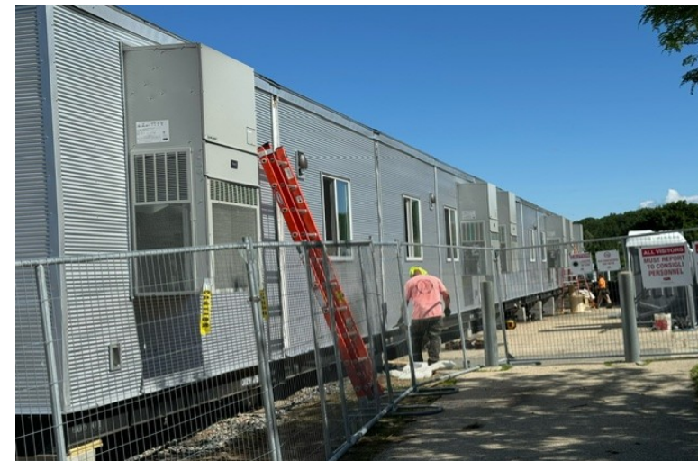
McDonough Modulares Being Set
