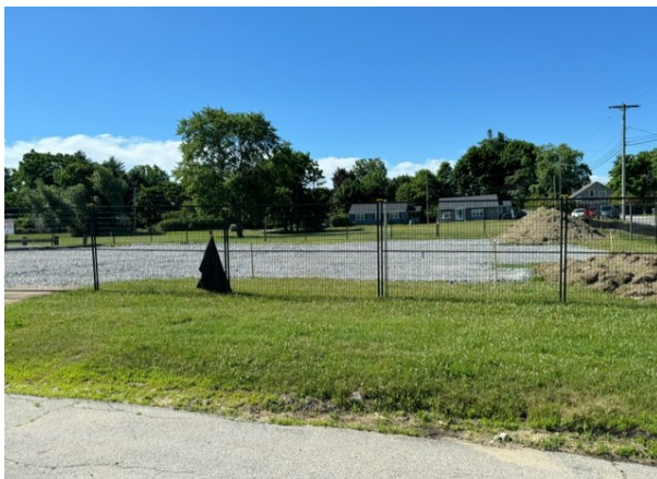
McDonough Parking lot Prep-work
