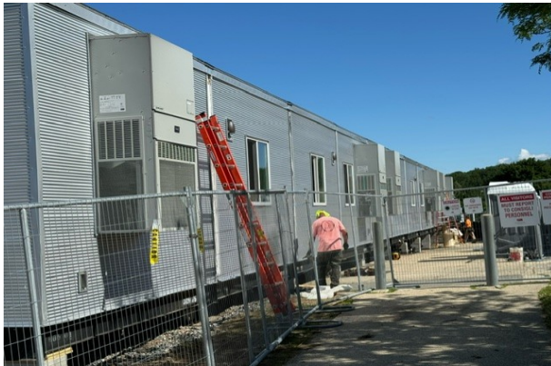
McDonough Modular Unit Set in Progress
