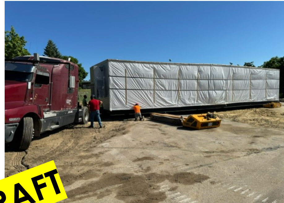
Southside Modulares Being Set
